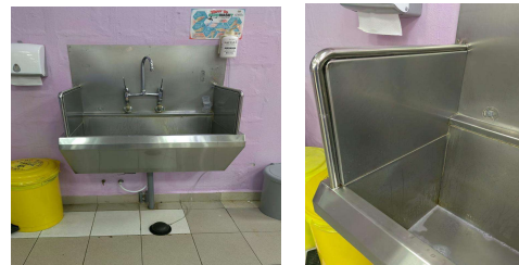
Figure 2. Clinical sink with partition to prevent water splash
